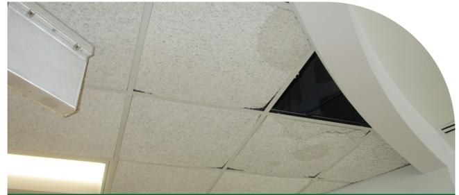
Pieces of the ceiling in Eagle Hill Middle School are warped and damaged due to leaking.
