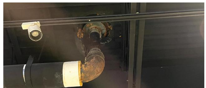
A pipe in the high school art wing is nearly rusted through due to consistent leaking from the roof.
